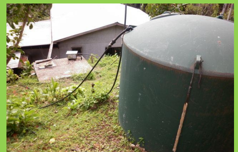
Concrete Well & Nura Tank
